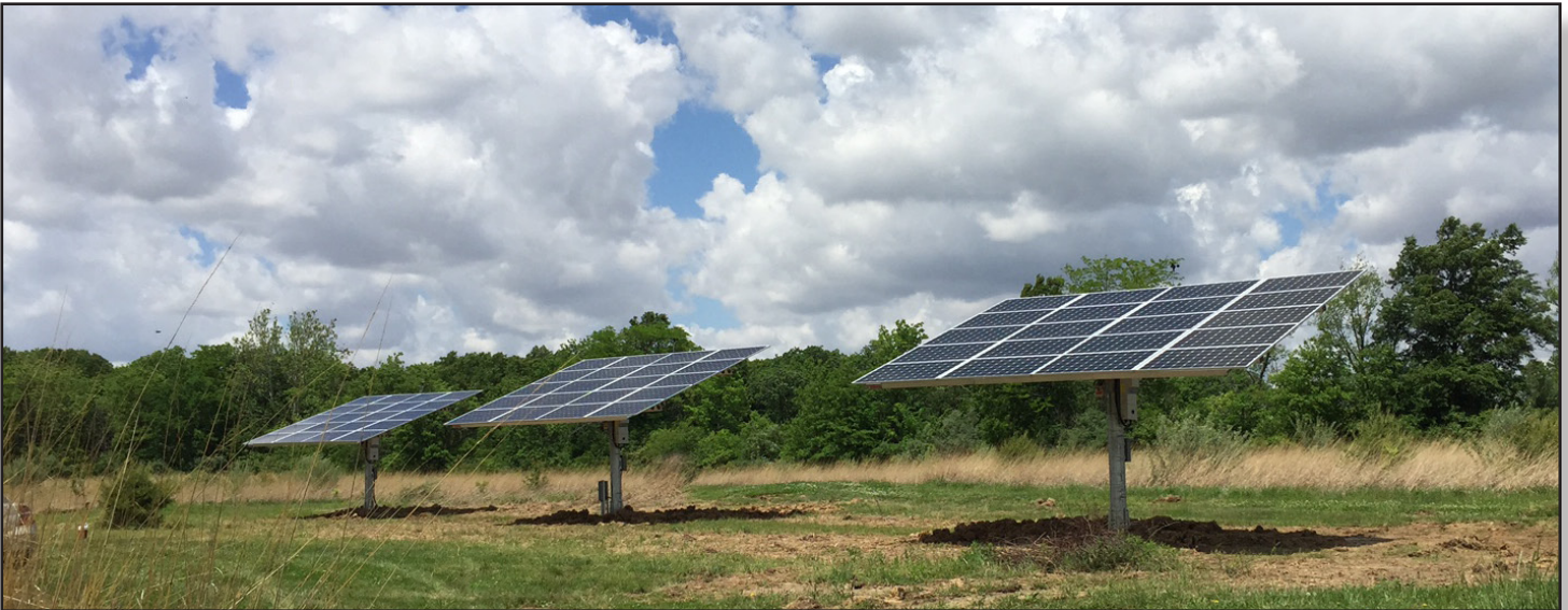
Three (3) 5.6 kW (DC) AllEarth Renewables Solar Trackers
