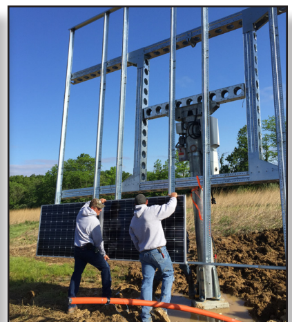
Installation of Solar Panels on Tracker
